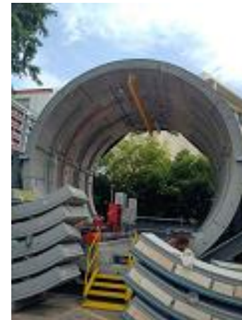
SAMPLE MOCK UP AT PROJECT SITE
