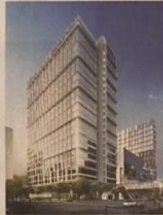
The 23-storey Junction City Tower - developed by Keppel Land and Myanmar's Shwe Taung Group - has Grade A office space with a net leasable area of about 33,400 sq m. PHOTO: KEPPEL LAND
